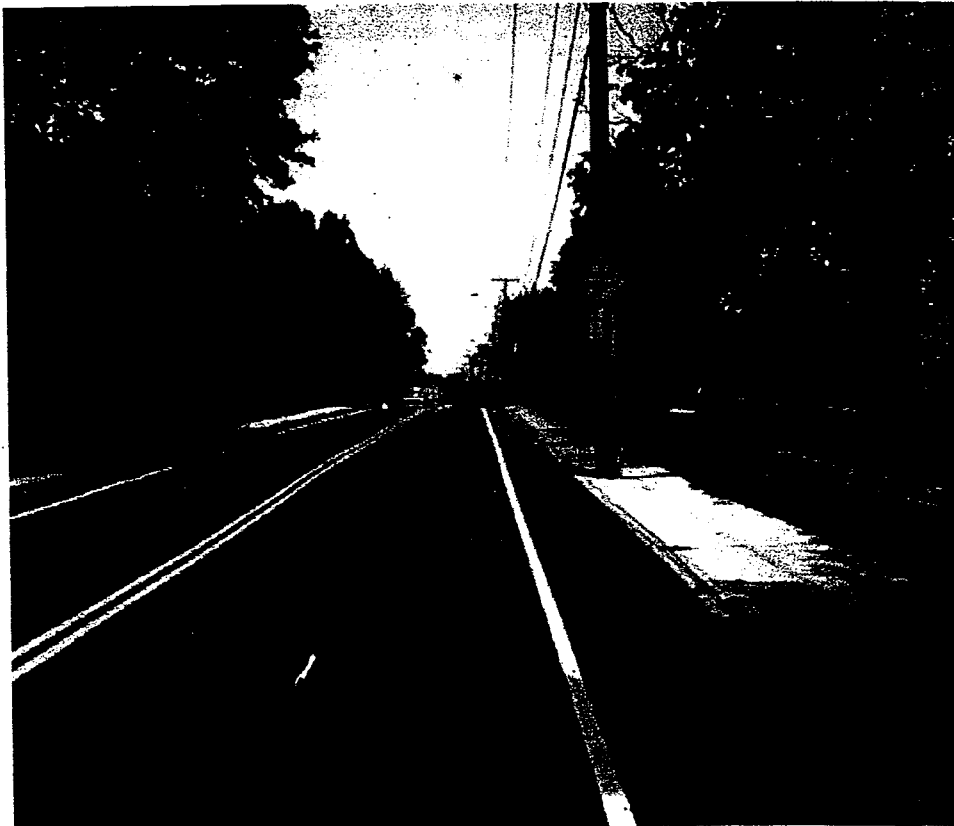
Figure 3.20: Sight Restriction Due to Vertical Curvature
