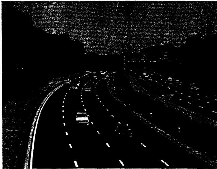
Figure 17.1: Typical Markings on a Freeway
